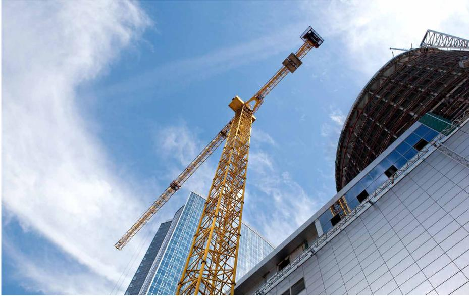
Depending on the model type, size, counter weights, and configuration of the crane, these cranes have maximum rated load capacities determined by the manufacturer. Typically the longer the boom length and greater the radius, the rated capacity is lowered or reduced.
