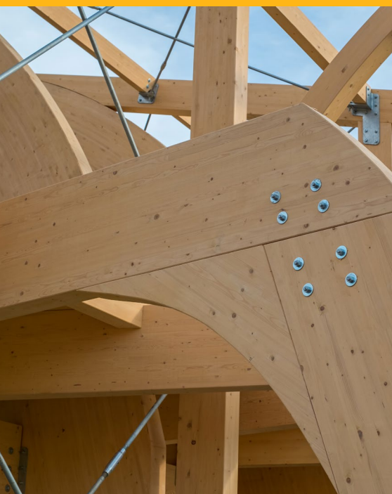
Detail of modern wooden architecture in glue-laminated timber (Glulam)
